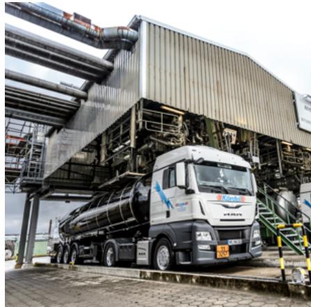
Safe truck loading.
