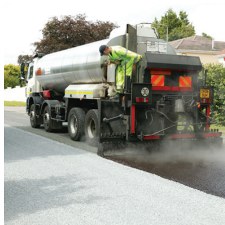
Bitumen emulsion surface treatment.
