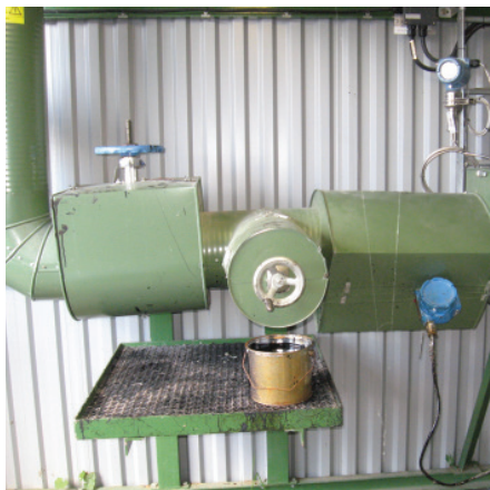
Bitumen sampling point.
